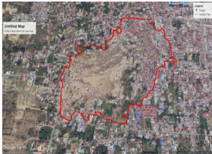
Figure 6. Post-liquefaction image of Petobo with damage outlined for assessing the earthquake's impact on the community.
