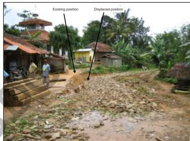
Figure 17. Creeping at village of Wangun 3, Bogor landslide area. There is a road surface displacement of 0.5 m from existing level position to a lower position
